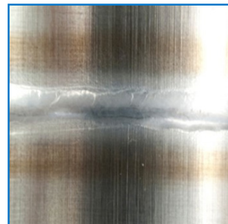
HEAT TINTS REMOVED
