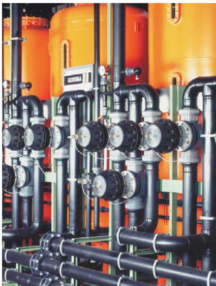
Waste water plant with PVC/PE components
