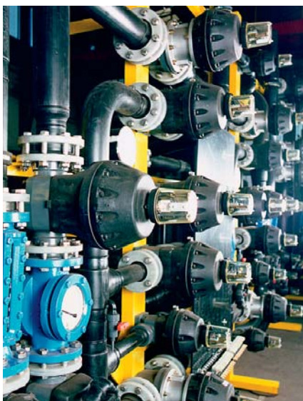
Waste water plant with PVC/PE components
