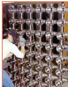
Steve welding CSI's first valve manifold, 1988
